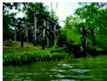
Disused coal loading facility at Tivoli
