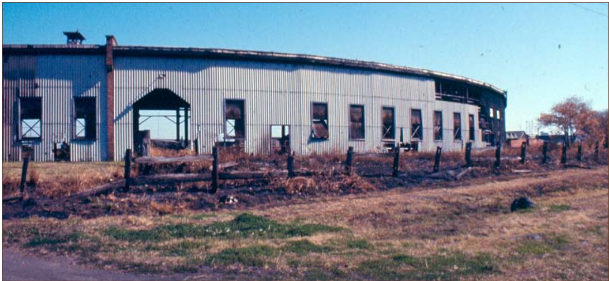
The Roundhouse shortly before it was demolished
