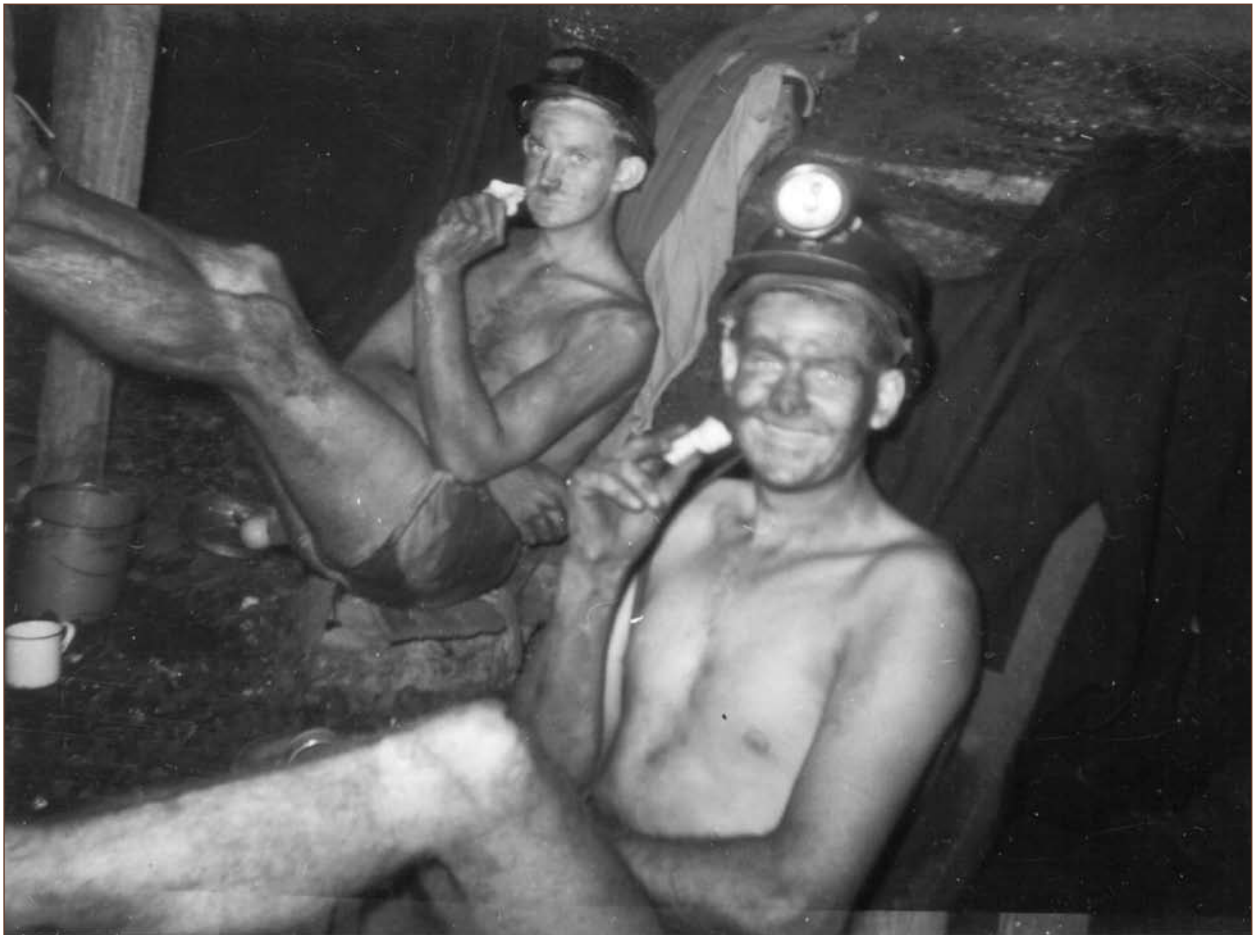
Photo 9: Crib time underground,
