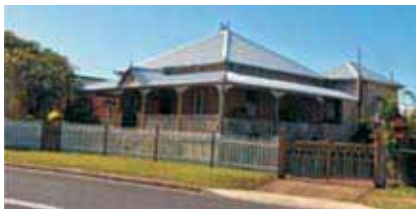
2 Ferrett Street, Sadliers Crossing
