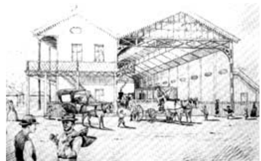
The first Ipswich Railway Station. Tattersall's omnibus has just got a passenger
