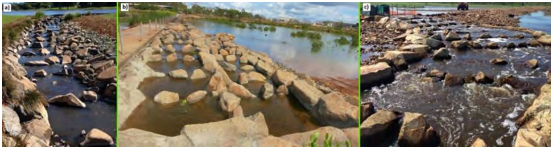
Figure 6. Nature like rock-ramp fishways: a) Full width (Gooseponds Ck, Mackay), b) Dog-leg (Lake Callemondah, Gladstone) c) Partial width (Tedlands Ck, Koumala)
