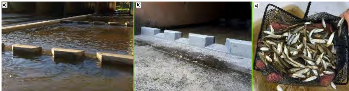
Figure 10. a) Retrofitting horizontal culvert baffles in operation under Paradise Road on Slacks Creek. Note: Nib wall to divert all base attraction flows down the fishway. Prior to remediating this barrier, the flow was spread out across four 2.4 m wide culvert barrels creating a shallow water surface barrier under base flow conditions. b) Horizontal baffles with the boxing recently removed c) Predominantly showing Juvenile sea mullet and striped gudgeon captured successfully ascending through the horizontal culvert baffle fishway at catch rates of 256 and 793 individuals per day respectively.
