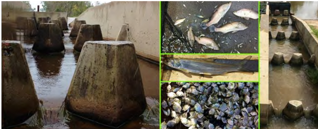
Figure 7. Concrete cone fishway on Boundary Creek, Koumala; showing fish successful at ascending, top to bottom; juvenile barramundi and empire gudgeon, giant herring & over one thousand juvenile banded scats & threadfin - silver biddy.
