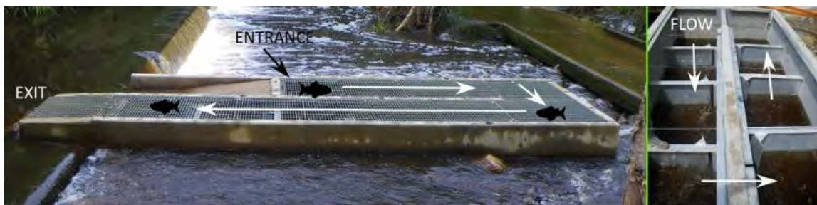
Figure 8. Showing a vertical-slot fishway on Waterpark Creek, Byfield. Note: The partial width nature and small entrance of vertical-slot fishways means it may be difficult for fish to locate the entrance.
