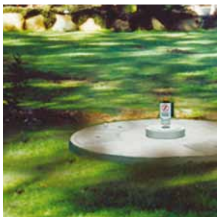
An operational septic system
