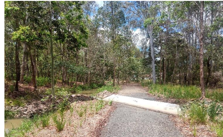
Reconstructed weir at Moodai Reserve – December 2022
