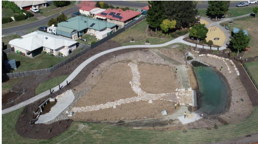
Sarah Drive Park Bioretention Basin during final stages of construction
