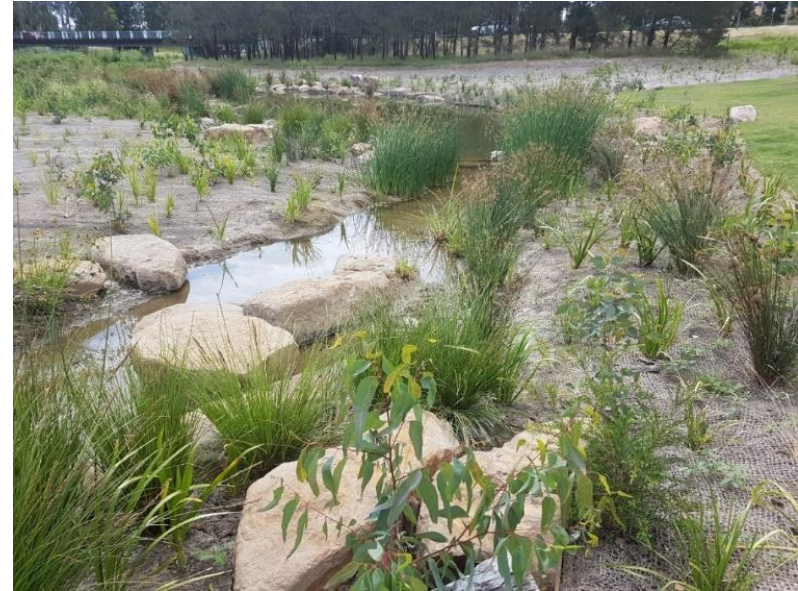
Downstream reach of Small Creek soon after completion
