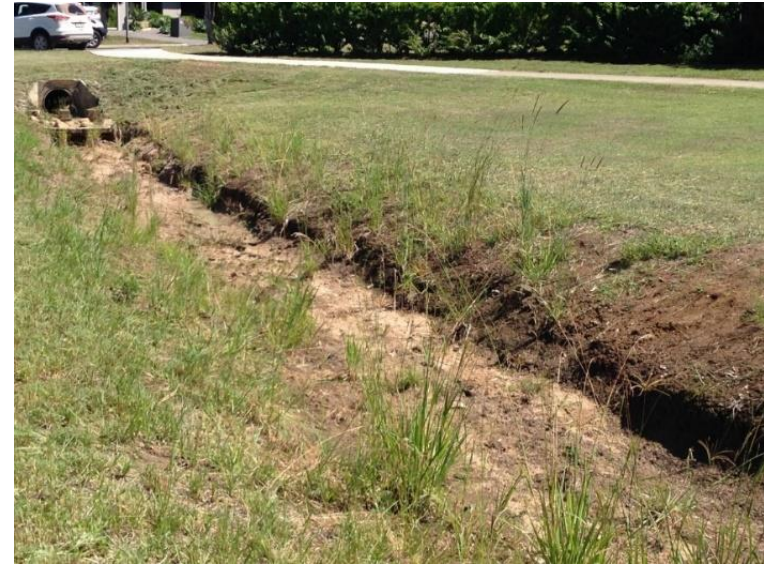
Headwall and channel prior to works being undertaken
