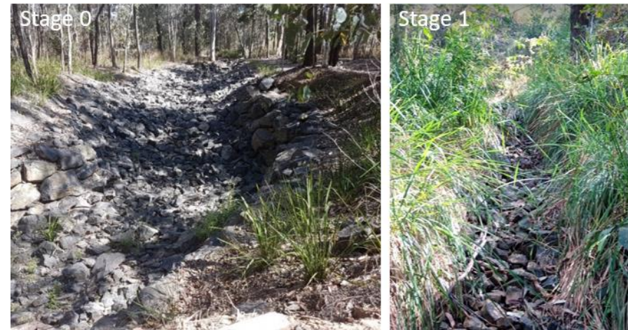
Ironpot Creek Stages 0 and 1, stabilising actively eroding gullies
