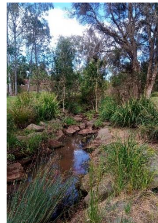
Pollard Park Channel Naturalisation (November 2022)
