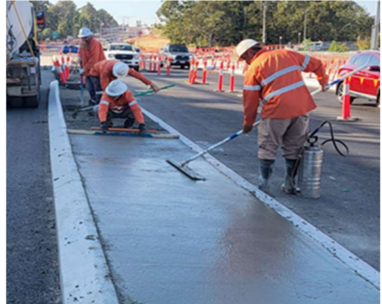
Centre median concreting Springfield Greenbank Arterial
