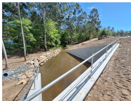
Stage 2 – Culvert, head and wing wall completion
