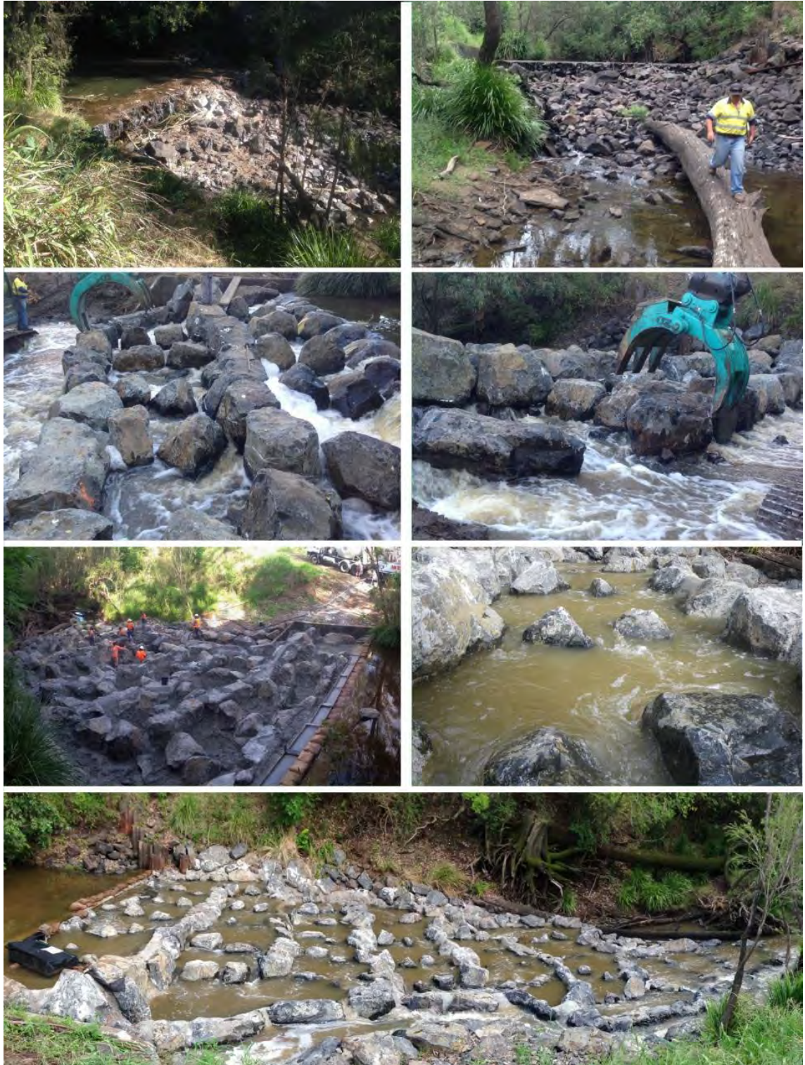
Figure 24. Berrys Weir fishway construction images
