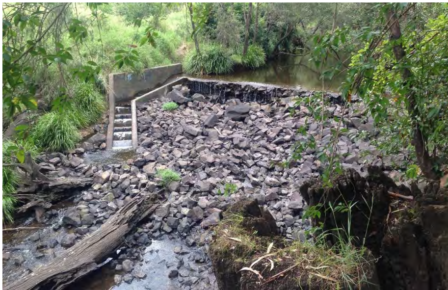
Figure 23. Berrys Weir fish barrier before remediation works, with relic north- American style fish ladder visible down left side of weir
