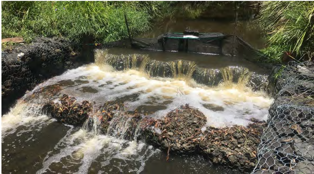
Figure 11. Image of fishway trap and wing wall assembly set above the Warrill Creek sheet pile weir
