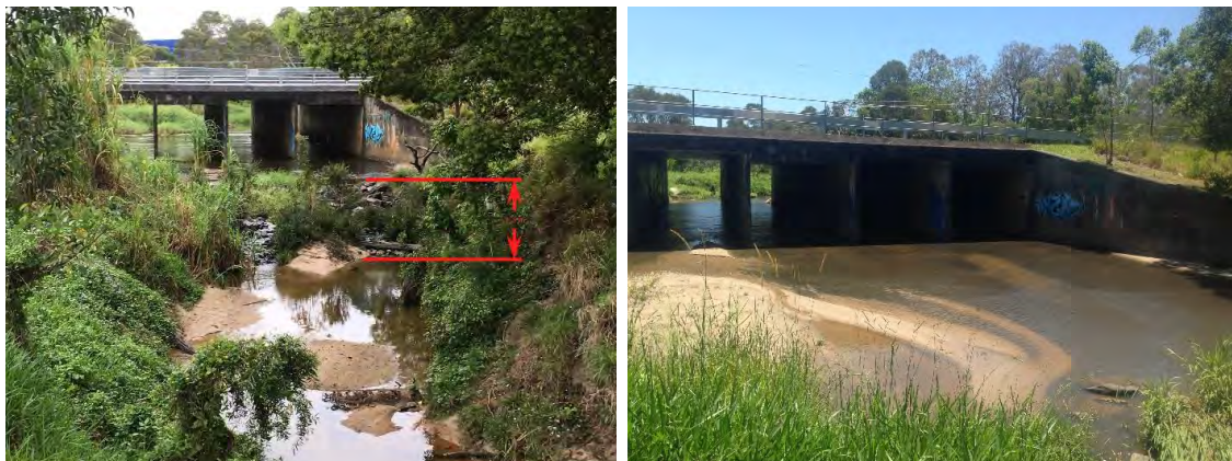
Figure 20. Left; showing the 1.3 m surface drop barrier off the downstream face of the culvert apron. Right; showing stream flow spread out across all four box culverts creating a shallow water surface barrier along the entire 50 m length of the structure. During stream flow events the culverts also created a flow velocity barrier.
