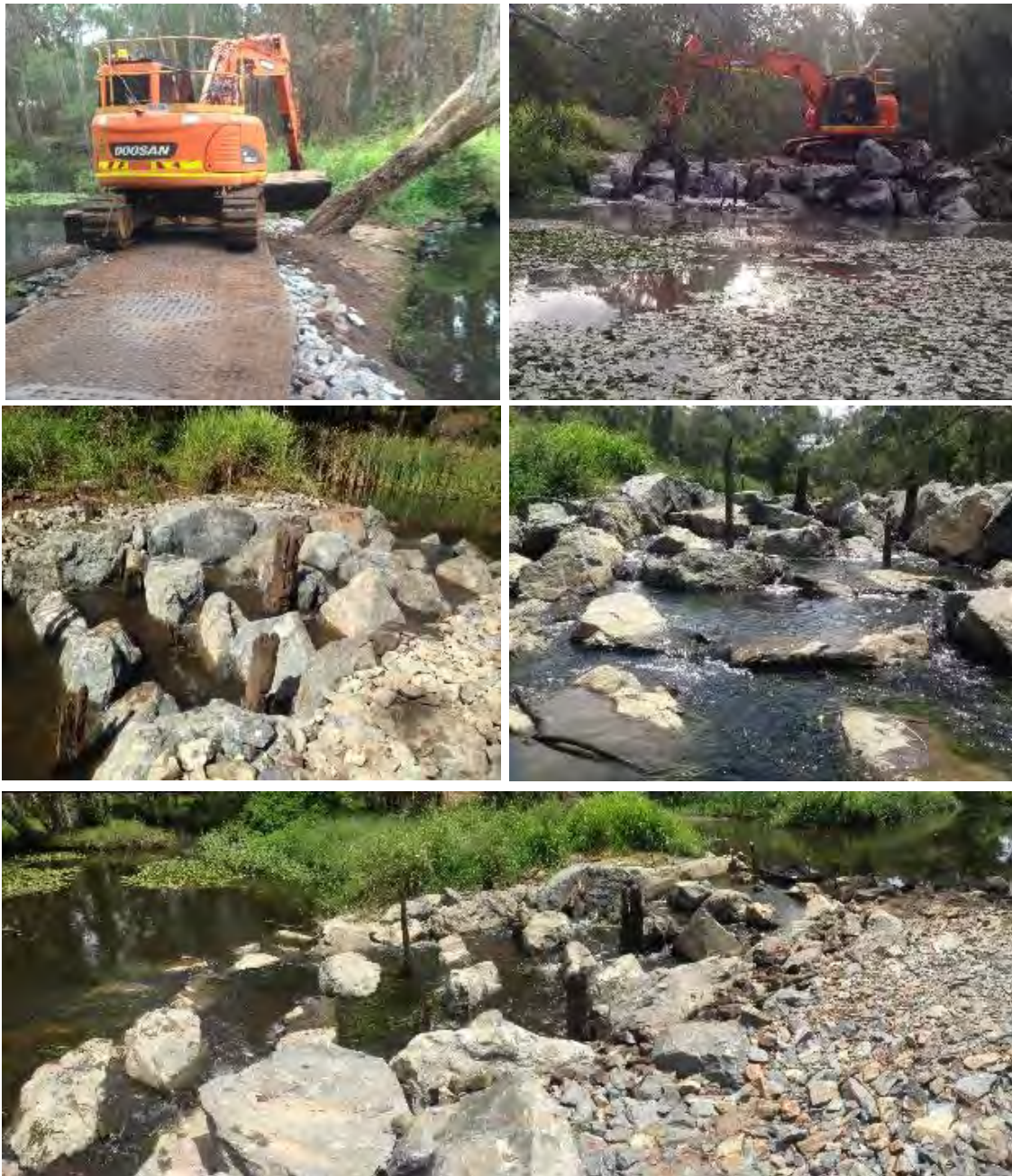
Figure 30. Showing construction images of Hilliards Creek fishway
