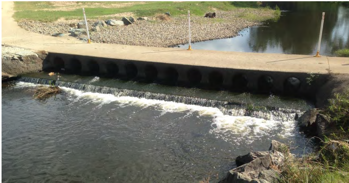
Figure 26. Showing Leitchs Crossing fish barrier prior to fishway construction
