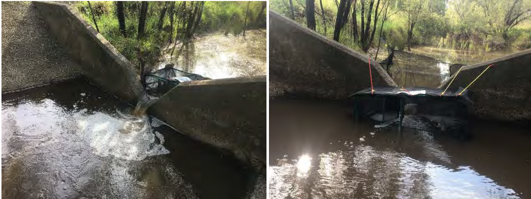
Figure 5. Fish trap set above the V-notch gauging barrier (left), and below the barrier (right)
