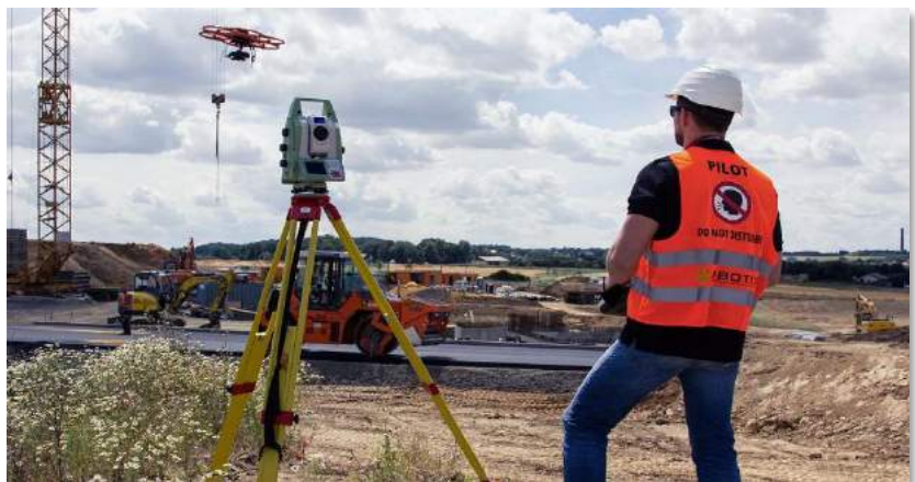
FIGURE 42: Drones can be used to undertake digital surveys for municipal infrastructure design.
