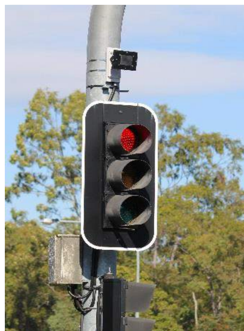
FIGURE 5: Traffic signals in Ipswich with radar technology to detect approaching vehicle speeds and adjust signal operations.
