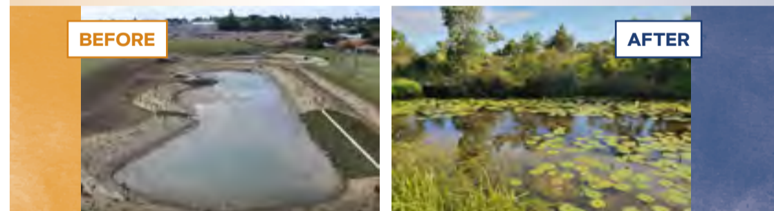
Constructing Wetlands – Jim Donald Wetland
