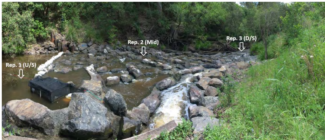
Figure 3. Fishway showing points of water quality readings which were upstream and downstream of the fishway, and also in the middle pool of the fishway
