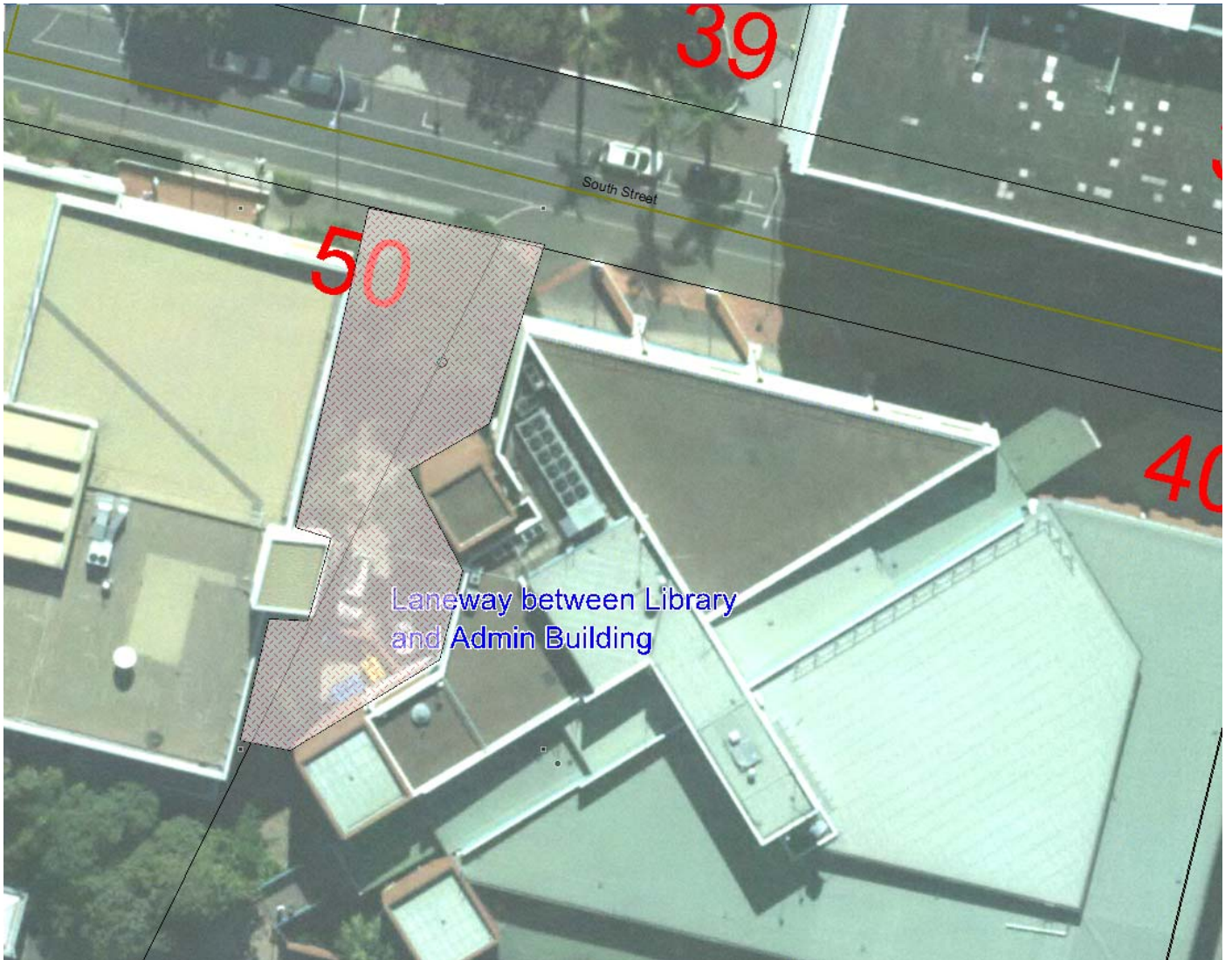
Laneway between Ipswich City Council Library and Administration building, 40-50 South Street, Ipswich
