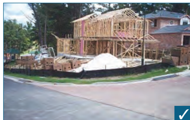
Effective on-site erosion and sediment control
