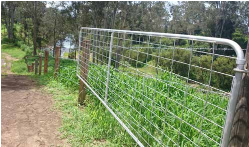
Seqwater installed fencing on the river bank rehabilitation site of this Mockers Road property in consultation with the owner
