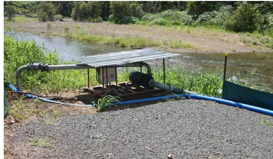
Ease of access to irrigation equipment in the event of river water rising can be considered as part of riparian works at each site
