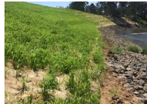
Before and after photos for a river bank rehabilitation site at Mockers Road, Fernvale
