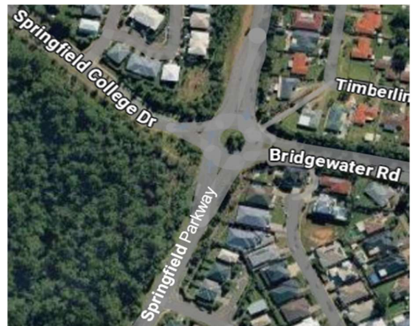
Work Location - Springfield Parkway College Drive Bridgewater Road Roundabout
