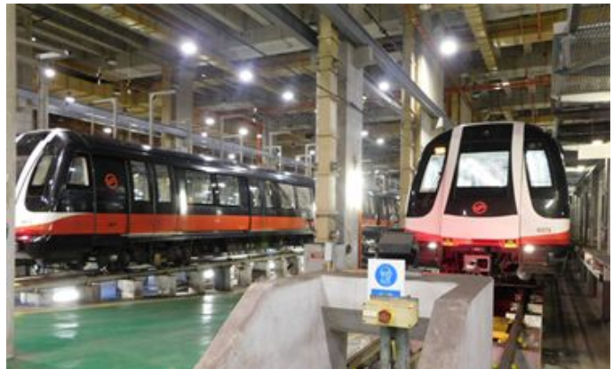
World's largest underground train depot (SMRT)
