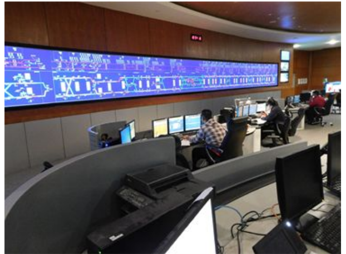
SMRT control centre for automated train operation
