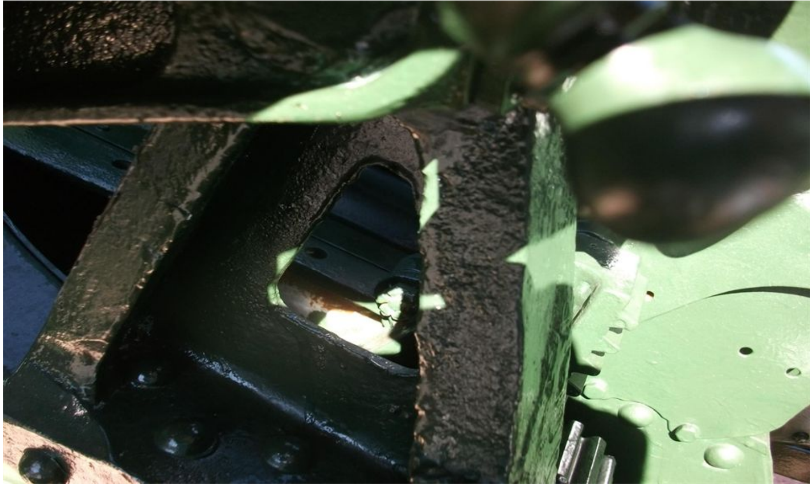
Barrel Left Side – The area in the center has not been painted and is starting to rust. Requires rust removal, re-priming and repainting.
