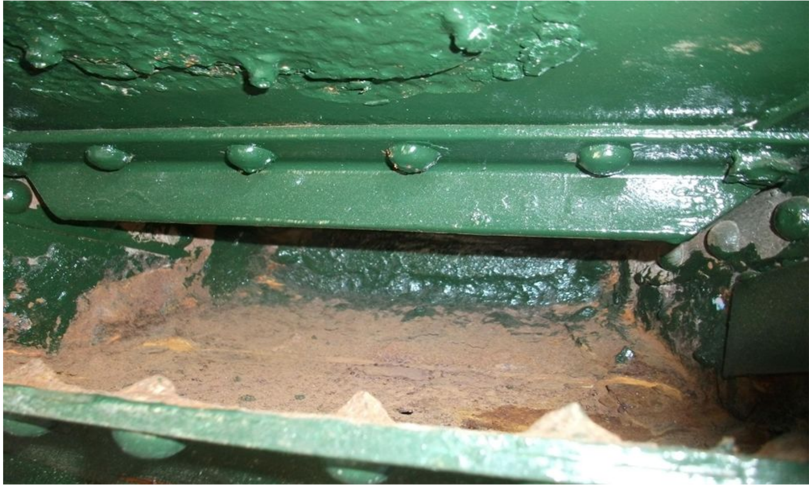
Rear Chassis Bottom Side – The top section of rusted out chassis can be seen. There is a very large area of unpainted surface which is already developing rust. Requires rust removal, re-priming and repainting.
