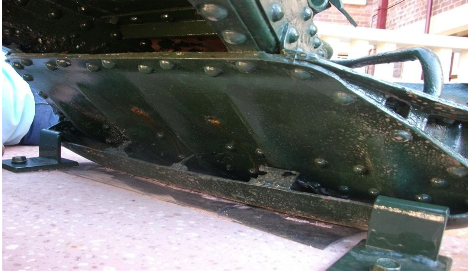
Rear Chassis Ground Level – Areas of past rust evident, new rust appearing, water settles in The base of chassis, rust on reverse side of chassis. Requires rust removal, re-priming and repainting.
