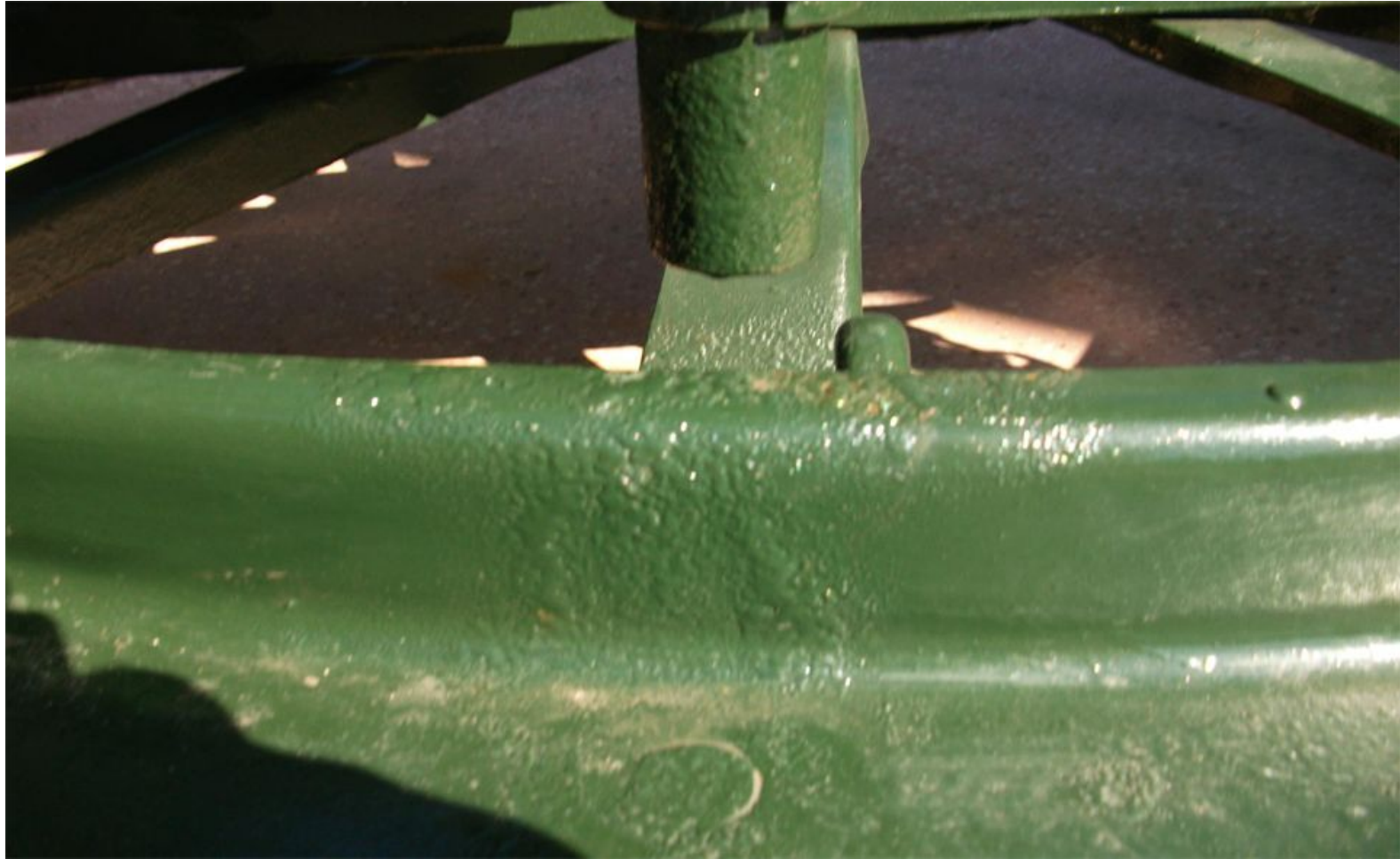
Traverse Mechanism Left Side – An example of rust area painted over and rust coming through.
