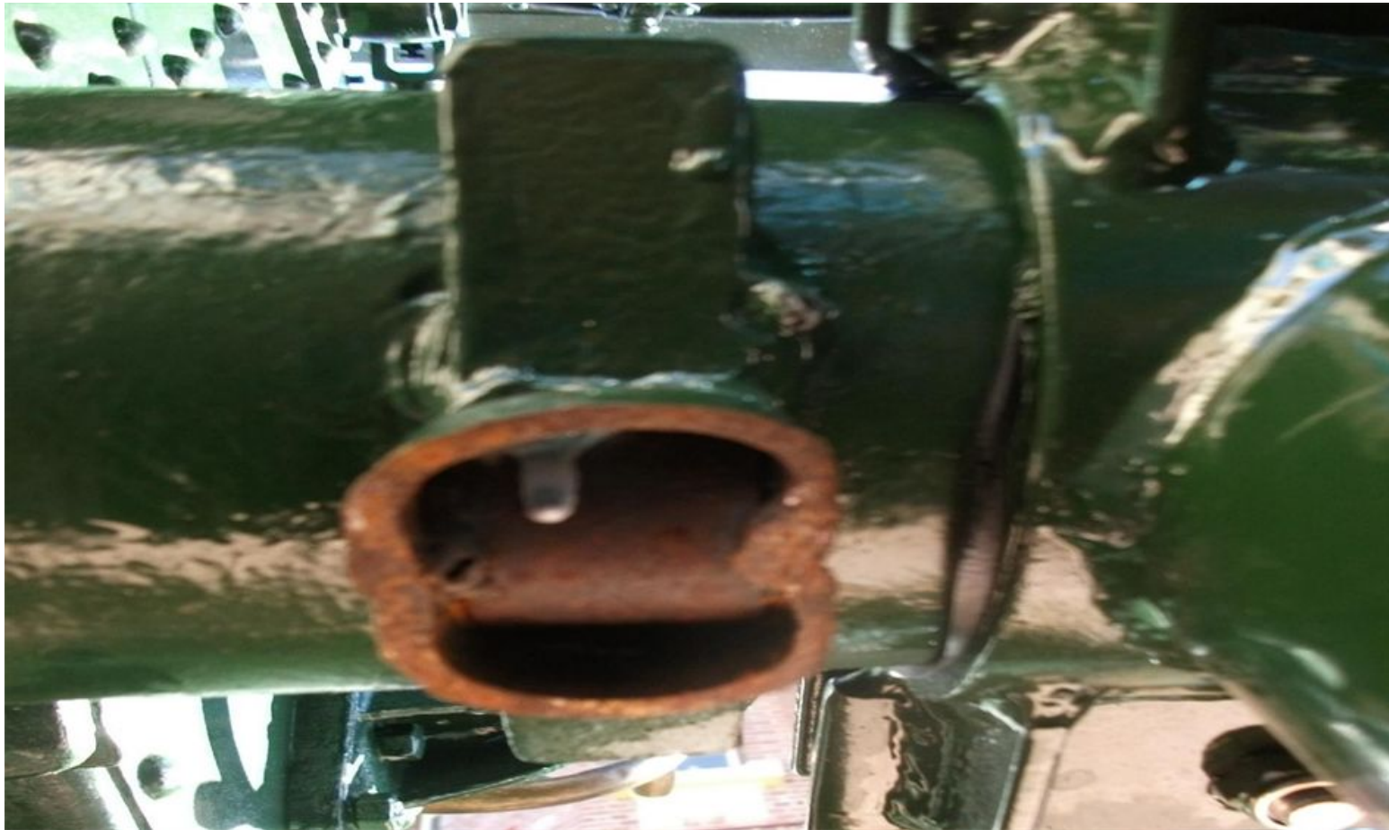
Left Hand Axle Casing underside – Something has been cut off the axle casing, it has not been primed or painted over and is now rusting. Requires rust removal, area sealed, re-priming and repainting.
