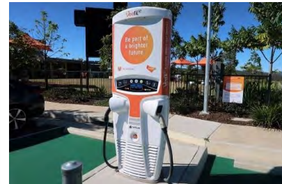
FIGURE 39: An EV rapid charging station recently installed at Yarrabilba in Logan City
