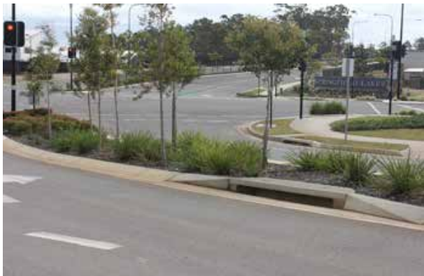
TMR is responsible for the stand-alone sub-surface drainage (gullies, manholes, inlets, outlets) of an intersection on the SCR where the sub-surface stormwater drainage is not connected to Local Government's stormwater drainage network.
