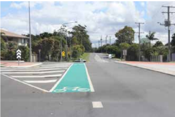
TMR is responsible for the entire carriageway through the intersection. (SCR)
