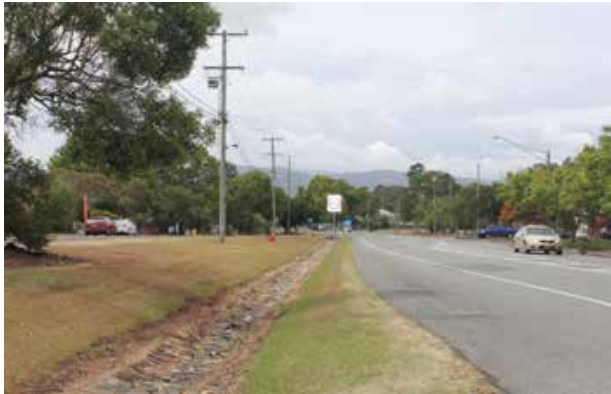
TMR is responsible for maintenance of the rock lined/concrete lined table drain.
