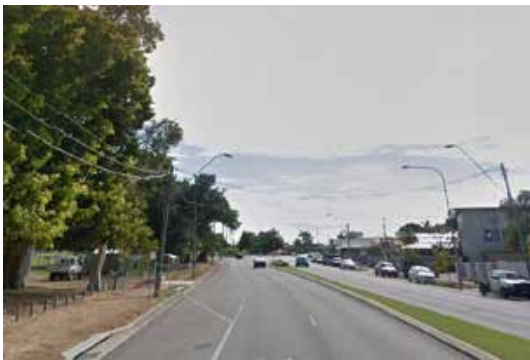
The edge line widening at the bus stop provides demarcation of traffic lanes that are the responsibility of TMR.
