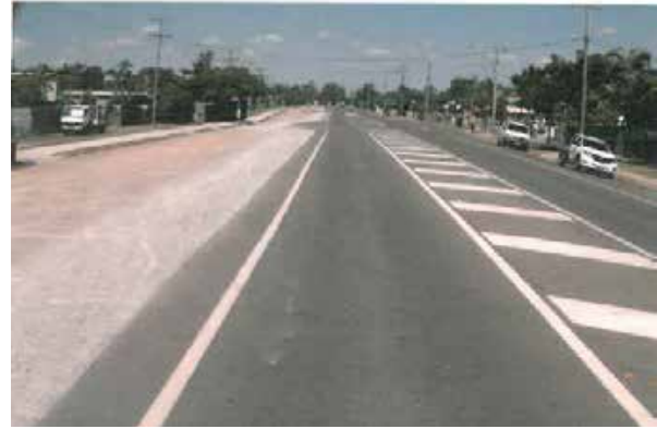
Given there is room for parking next to the kerb and channel, Local Government is responsible for the replacement of the kerb and channel at the end of its serviceable life.
