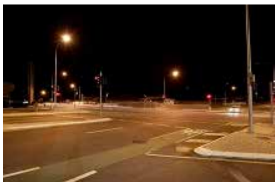
In the case of a local road with an extensive length of road lighting, the interface zone is to be agreed between Local Government and TMR. The costs of operating road lighting within the zone is met by TMR.
