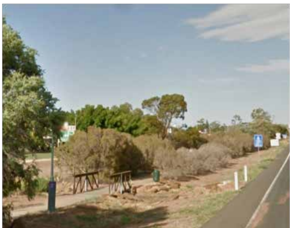
TMR is responsible from the carriageway to the back of the table drain. Local Government is responsible for the footpath from the back of kerb to the property alignment, including the footpath bridge structure.
