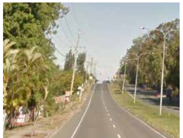
As there is insufficient space to park next to the kerb and channel, TMR is responsible for replacement of the kerb and channel at the end of its serviceable life.
