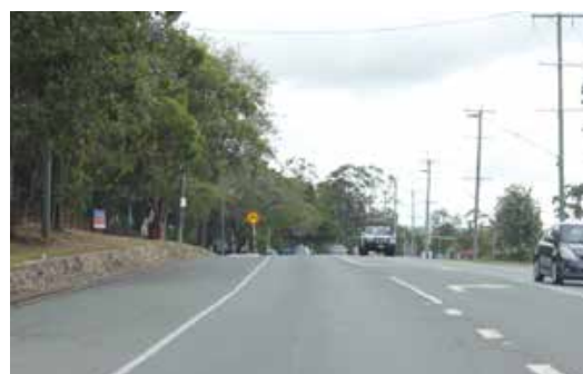
The edge line provides demarcation between the through traffic lane and the parking lane. Responsibilities for parking lanes are discussed in Module 3.
