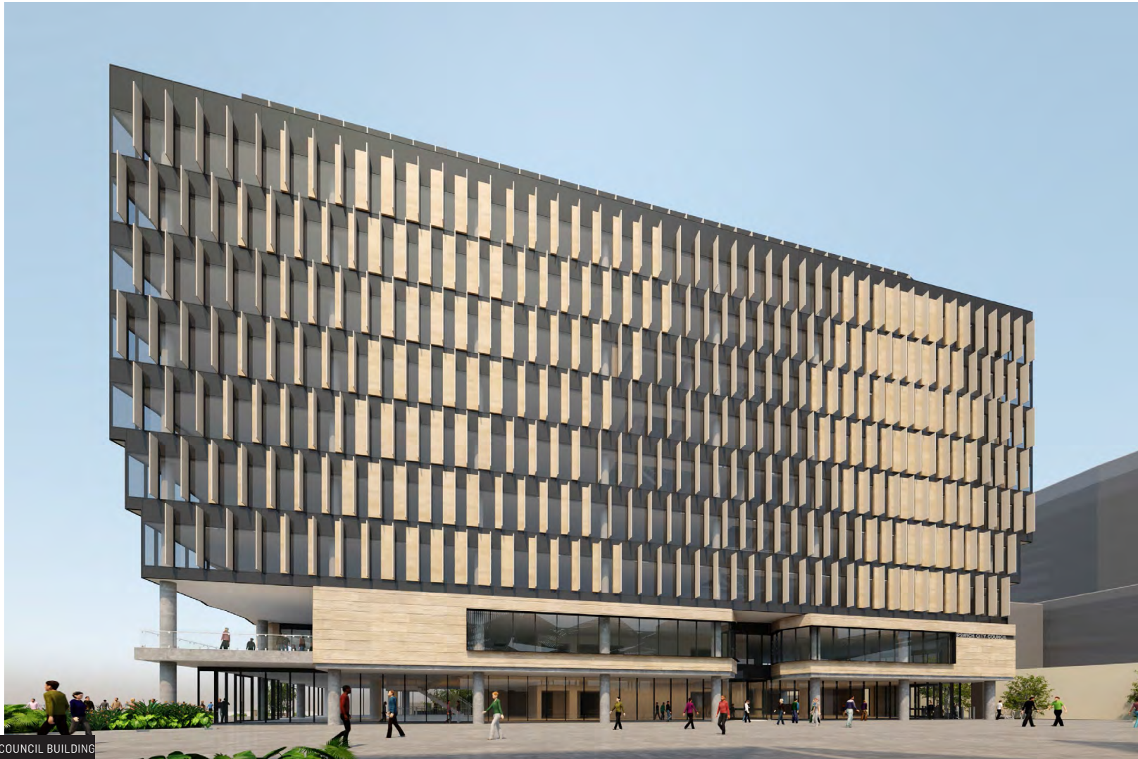
ICC IPSWICH CITY COUNCIL BUILDING
