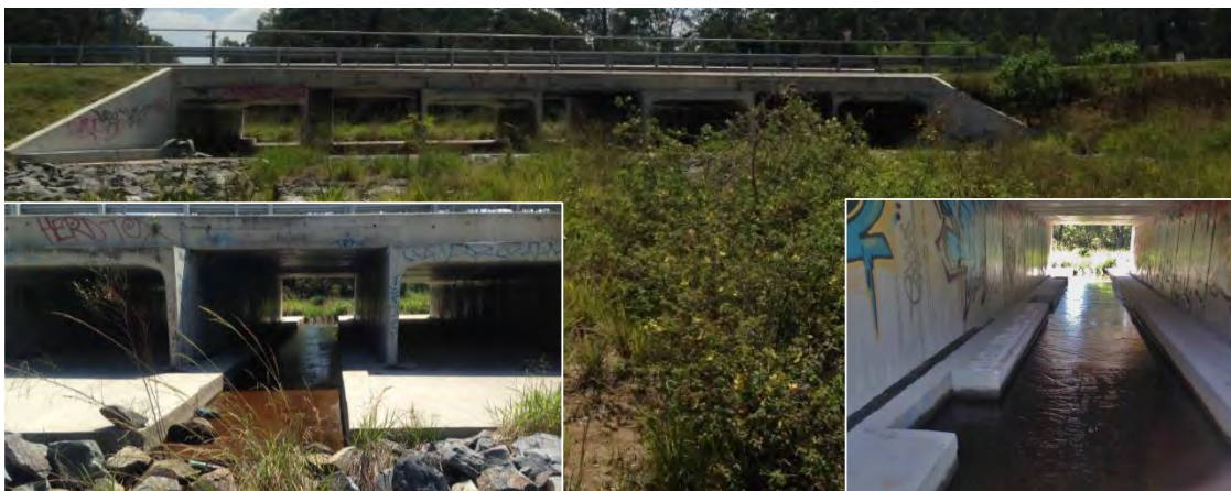
Figure 19. Culvert crossing conforming to Accepted Development requirements. Note: Low flow channel and wall roughening.
