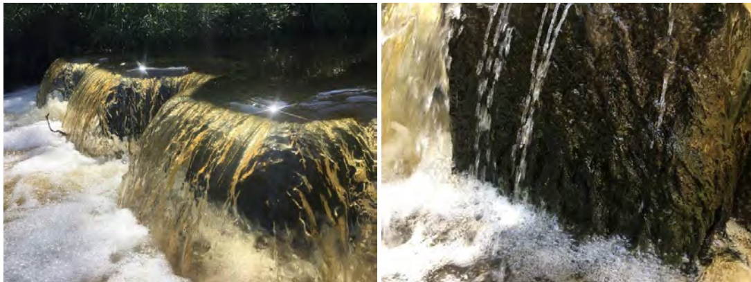
Figure 10. Close up image of the Warrill Creek sheet pile fish barrier (left), and close up of sheet pile surface showing roughness and algae used by striped gudgeon and eel sp. to climb this barrier (right).
