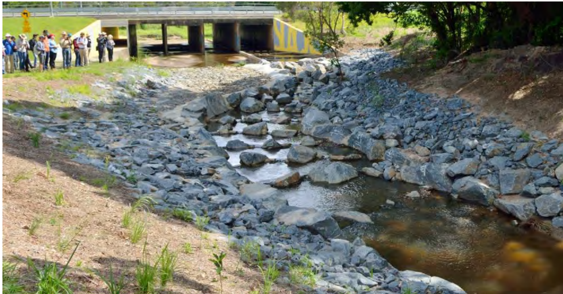
Figure 15. Showing one of the four priority ranked barriers remediated as part of this project; Slacks Creek, (Paradise Road) 17 ridge rock-ramp and horizontal culvert baffle fishway (photo courtesy of Leo Lee).
