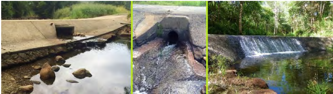
Figure 4. Left to right: Culvert causeway displaying a water surface drop, shallow water surface (through culvert and on apron) and velocity barrier (during medium- high flow conditions) exacerbated due to a culvert diameter <60% of stream width; Pipe causeway displaying velocity and behavioural barriers (dark shadows/insufficient lighting in pipe) and water surface drop barrier.
