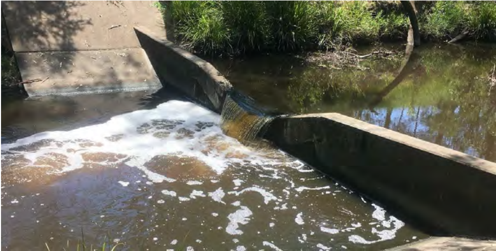
Figure 16. V-notch gauging station weir identified approximately 600 m upstream of sheet pile barrier
