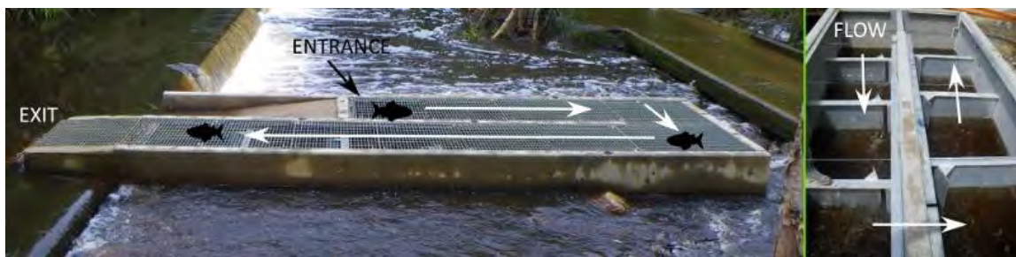
Figure 8. Showing a vertical-slot fishway on Waterpark Creek, Byfield. Note: The partial width nature and small entrance of vertical-slot fishways means it may be difficult for fish to locate the entrance.
