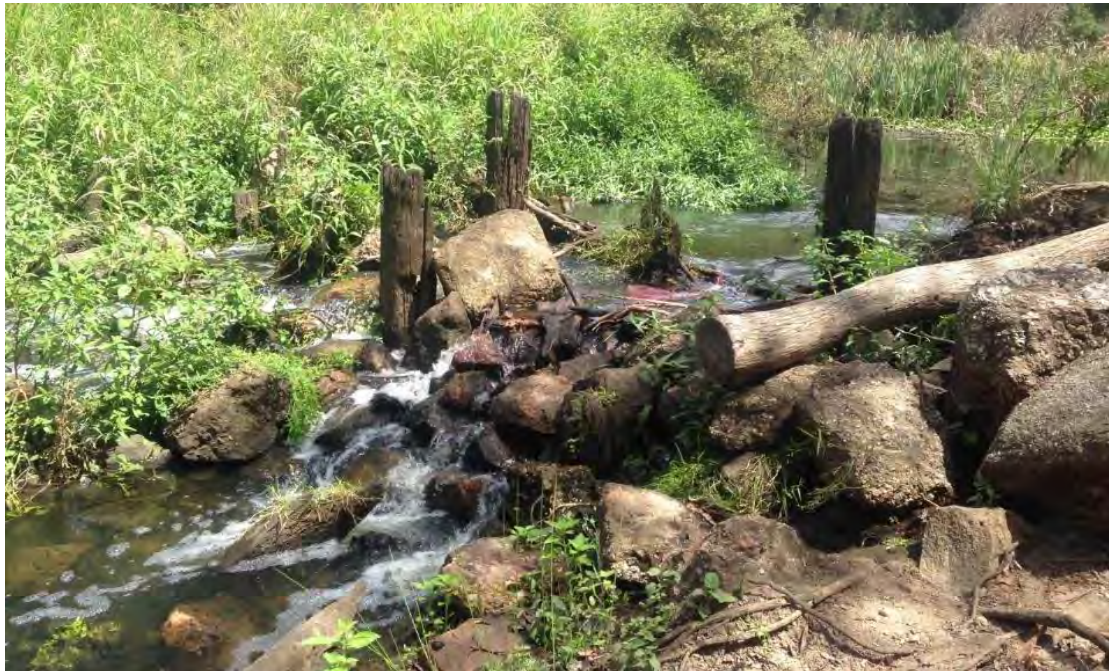
Figure 29. Showing the Hilliards Creek weir prior to fishway construction.
