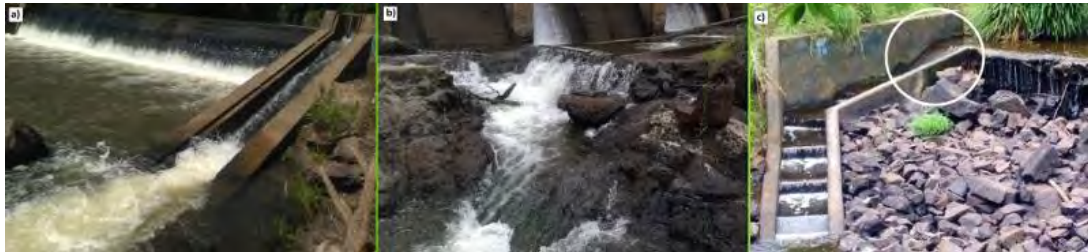
Figure 3. Showing northern hemisphere 'salmonid' style fishway designs exhibiting hydraulic conditions in excess of the swimming abilities of most native freshwater fish species. a) Denil fishway located on Luscombe Weir (Albert River, QLD) showing steep gradient and excessive velocities (note baffles removed). b) Showing the bottom section of the Mt Crosby weir pool and weir fishway (Brisbane River). Note the inadequate fishway entrance with excessive turbulence associated with the large water surface drop and shallow entrance pool and c) Pool and weir fishway located on the Bremer River (Berrys Weir). The exit of this style of fishway has a 600 mm high drop and velocities during base flows of 3.3 m/sec.
