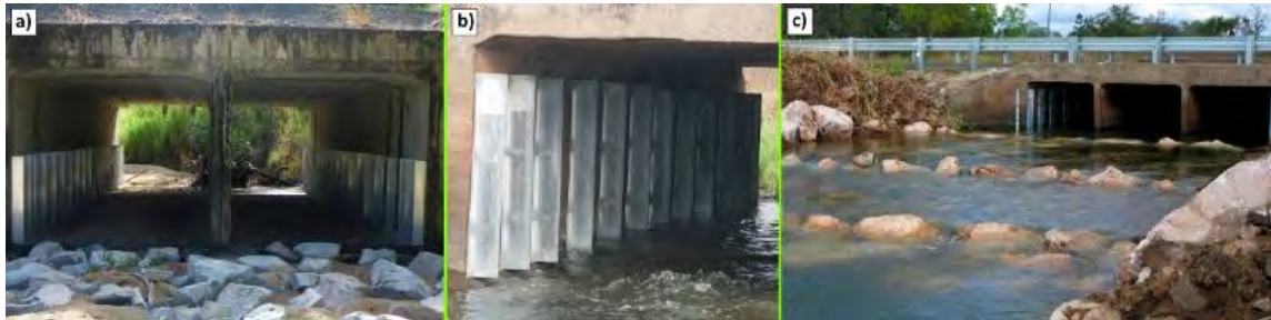
Figure 9. a) Vertical culvert baffles with scour protection (Aims Rd, Townsville) b) Close up view of vertical baffles retrofitted to a culvert c) Vertical baffles in conjunction with a rock-ramp fishway (Sheepstation Creek, Ayr).
