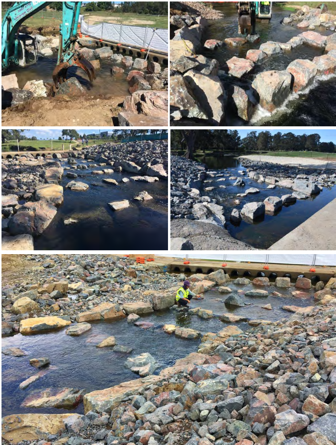
Figure 27. Showing during and post construction of Leitchs Crossing fishway
