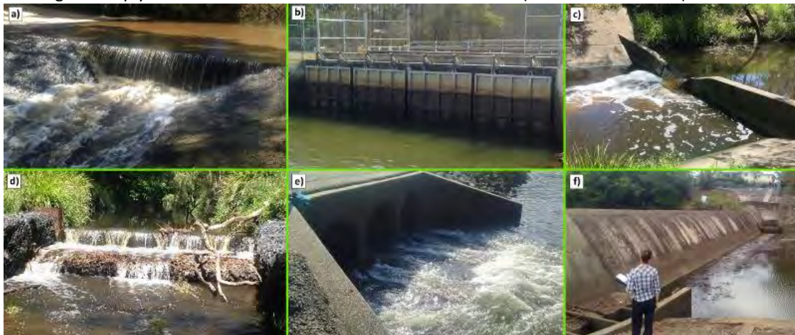
Figure 2. Barrier structures: a) Road causeway & concrete apron (Elimbah Ck), b) tidal floodgates (Behm Ck), c) V-notch stream gauging weir (Warrill Ck), d) Sheet pile and gabion basket weir (Warrill Ck), e) pipe culvert causeway (Albert River) and f) Tidal barrage (Caboolture River).
