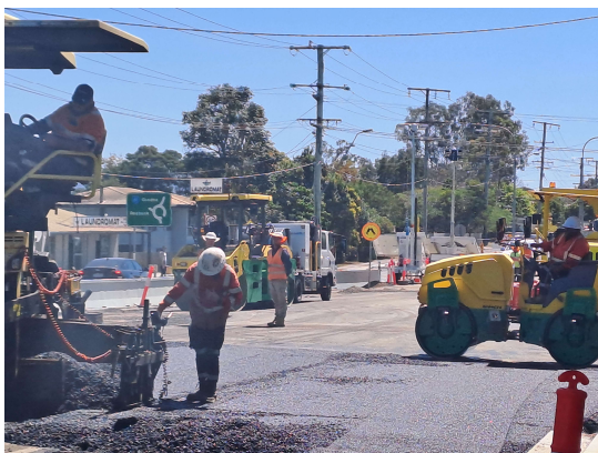
Asphalt laying works Redbank Plains Road
