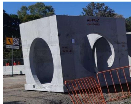
Stormwater drainage to be installed under Redbank Plains Road
