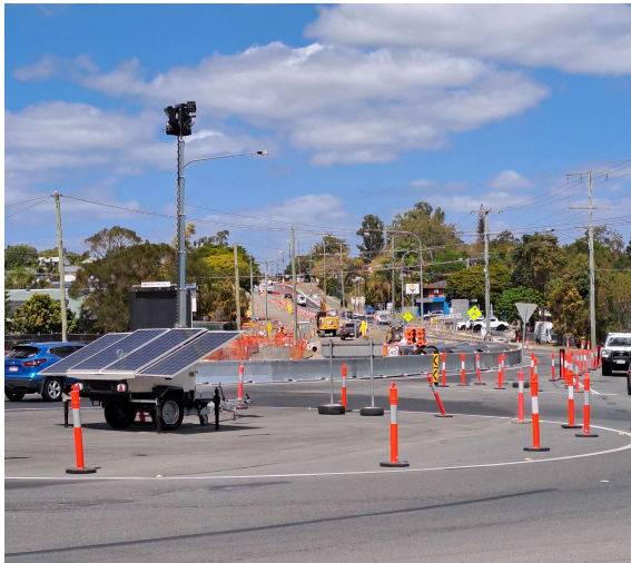
Redbank Plains Road construction from Kruger Parade
