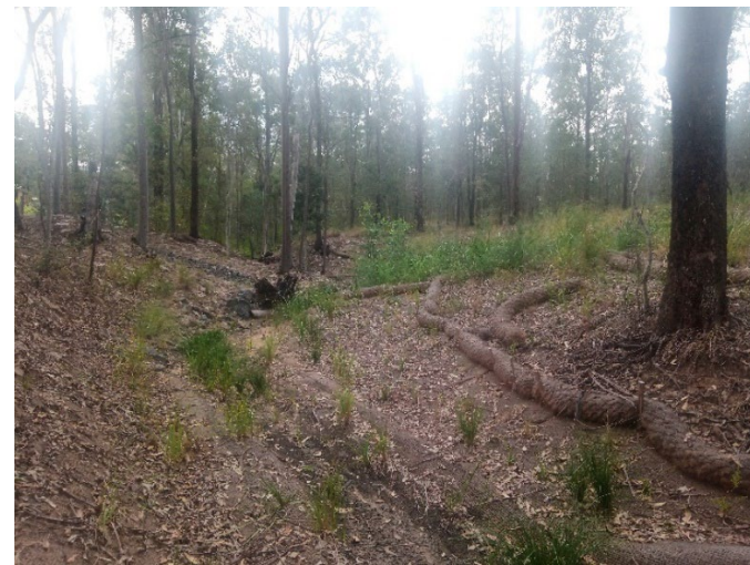
Ironpot Creek Stages 2, stabilising actively eroding gullies
