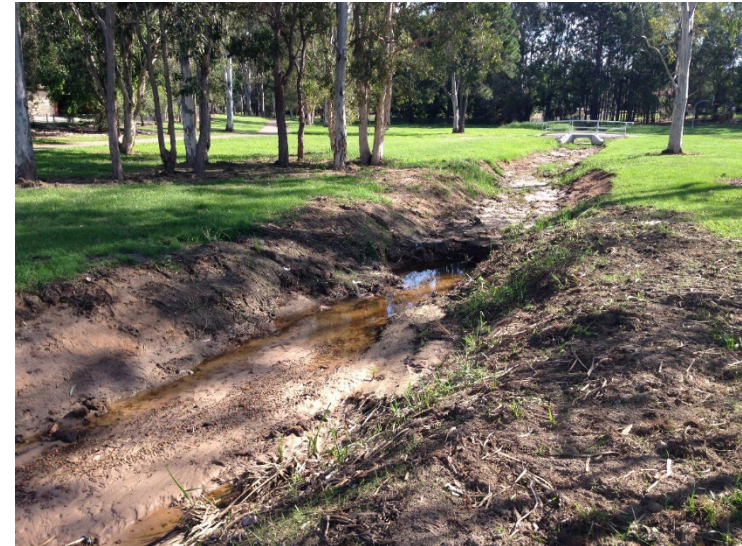
Erosion problems prevalent in Pollard Park pre-works contributing to elevated sediment and nutrient exports from the site
