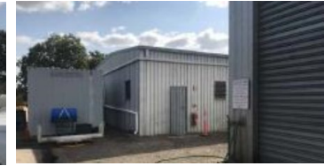
STORAGE SHED (B)
