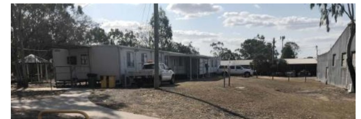
DEMOUNTABLE OFFICES (D, E)
