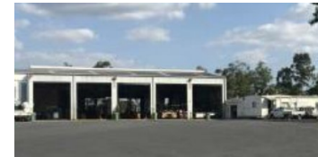
WORKSHOP BUILDING (A)
