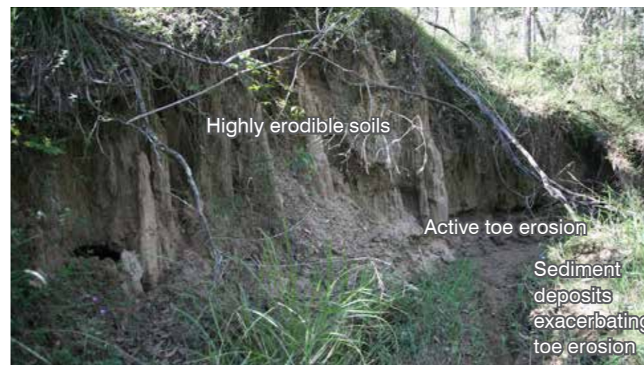
Figure 9. Active erosion occurring in the Upper Corridor
