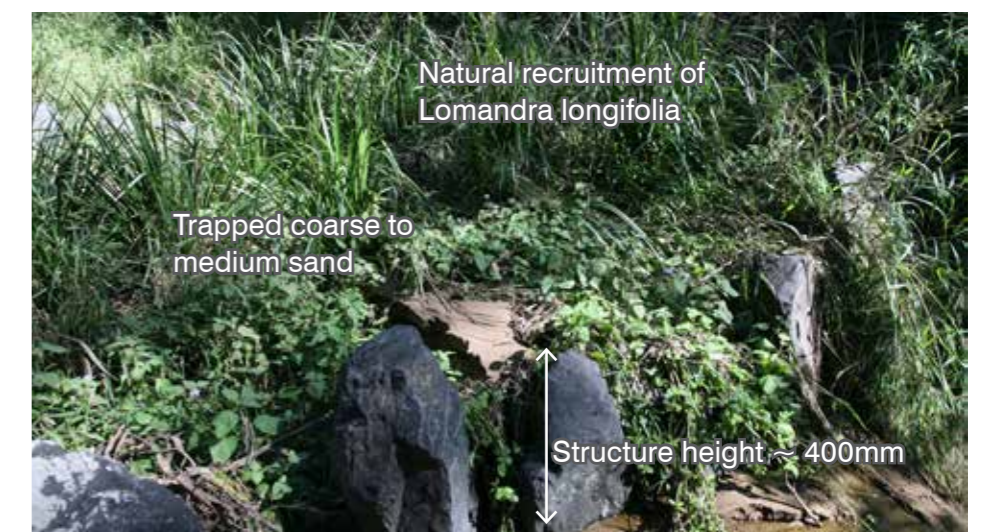
Figure 22. Photo of current sediment trapping upstream of Wairuna Court
