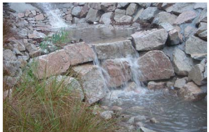
Plate 2: Use of rock chutes to improve waterway condition - Lilac Street waterway restoration (Image: AECOM)
