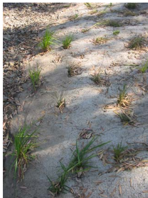
Plate 3: Geotextile materials require planting holes to be cut and regularly adjusted to allow vegetation to establish successfully.
