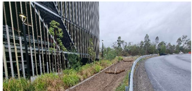
Stage 3- Core Logs Centenary Motorway Exit 32 off ramp
