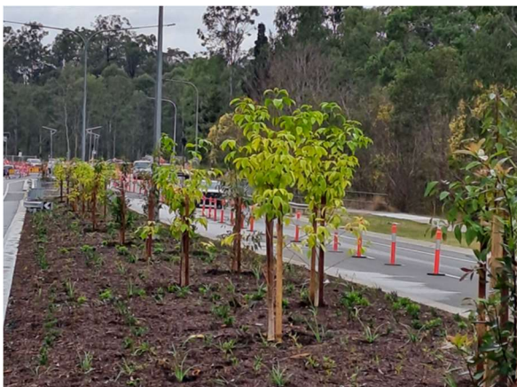
Stage 1 - Landscaping Springfield Greenbank Arterial
