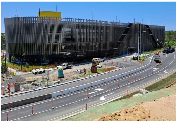
Stage 3 - Exit 32 construction
