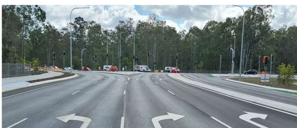
Stage 1 - Springfield Parkway Springfield Greenbank Arterial intersection
