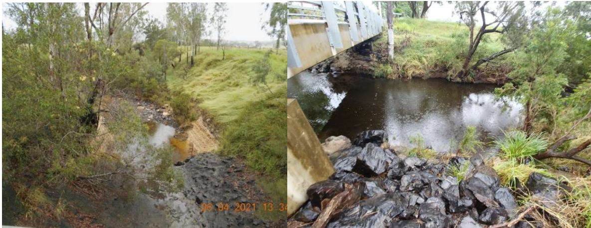
Figure 21. Banks around large bridges (left: Schmidt's Bridge – Grandchester-Mt Mort Rd, right: Franklyn vale Rd) reinforced with large rocks and concrete. Images: R. Grieger
