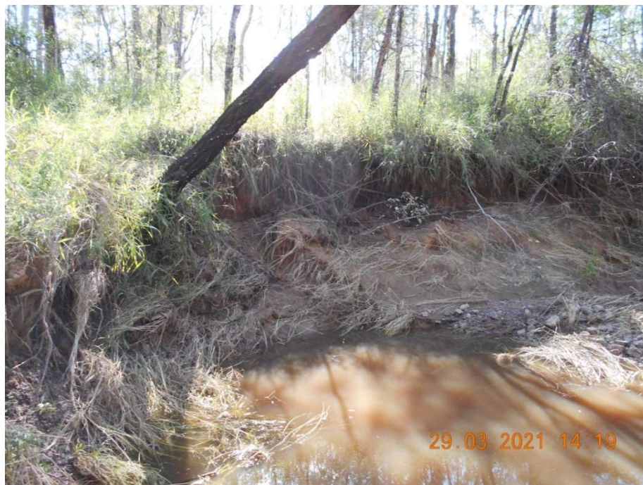
Figure 20. Erosion following a small blocked culvert at one creek crossing. Image: R. Grieger
