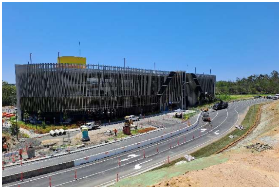
Centenary Motorway Exit 32 off ramp
