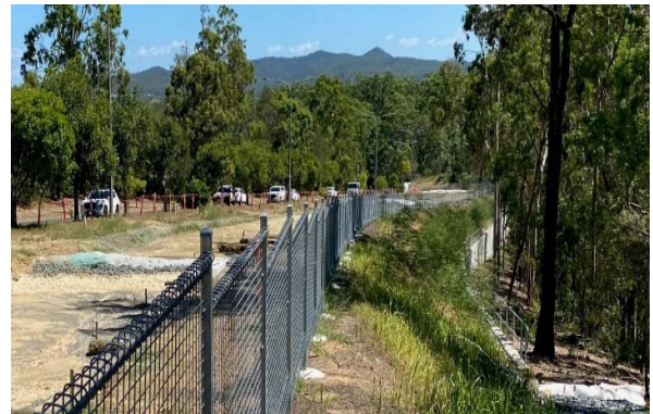
Eco blanket used to reinstate disturbed areas
