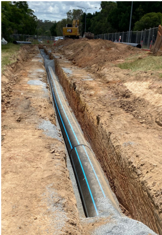
Installation of new water main.
