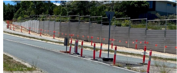
New retaining wall at Springfield College Drive
